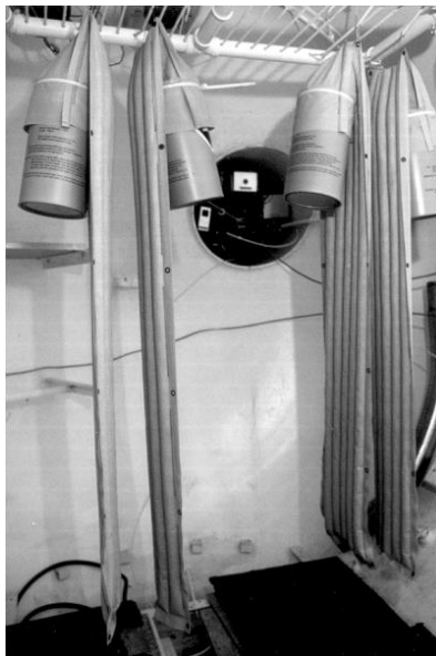
Figure 3.7.5 Lithium Hydroxide cannisters attached to Battelle Curtains [17]
